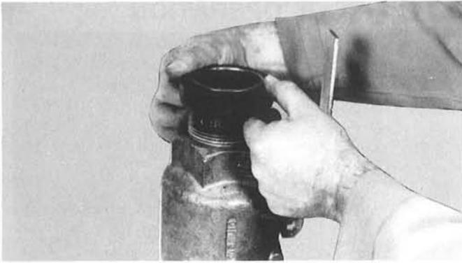
4. Install gasket over grooved end of Mechanical Tee/Valve Assembly unit as shown, being sure gasket lip does not overhang the end of the pipe.
